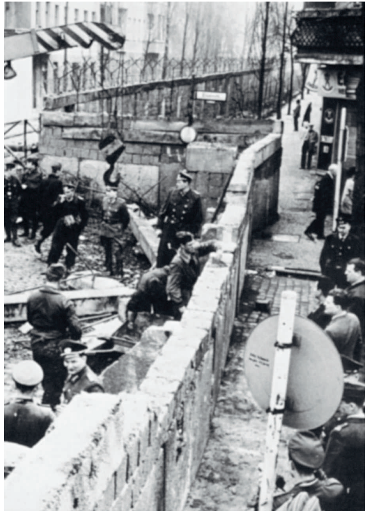
37 Berlin, Germany: Building the Berlin Wall, 1961
