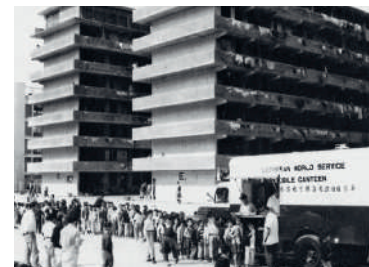
24 The design of the buildings recognized the needs of such a large-scale neighborhood: shelter was not the only component. The ground floor was left open for community use, providing space for shops, workshops, and services.
