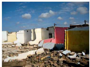
38 Destroyed houses in Errahma Bidonville
