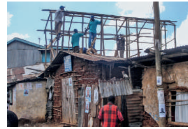
4 Small one-story, single-room residential shacks are pieced together out of wattle and daub walls (tree branches with clay construction), found objects, and rusted corrugated metal roofs. These dwellings house up to eight people and do not have basic living infrastructure such as running water or toilets. Kibera itself does not have a sewerage system.
