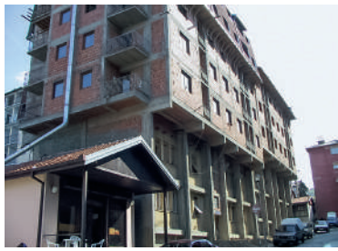
6 Roof extension mushrooming out over an existing building: "Russian pavilions," Karaburma, Belgrade
