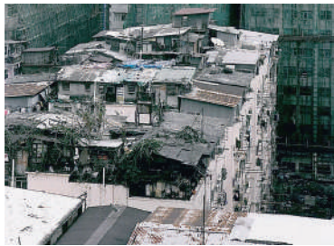
46 Illegal roof-top constructions, Tai Kok Tsui Area, Kowloon, from Rufina Wu and Stefan Canham, Portraits from Above: Hong Kong's Informal Rooftop Communities
