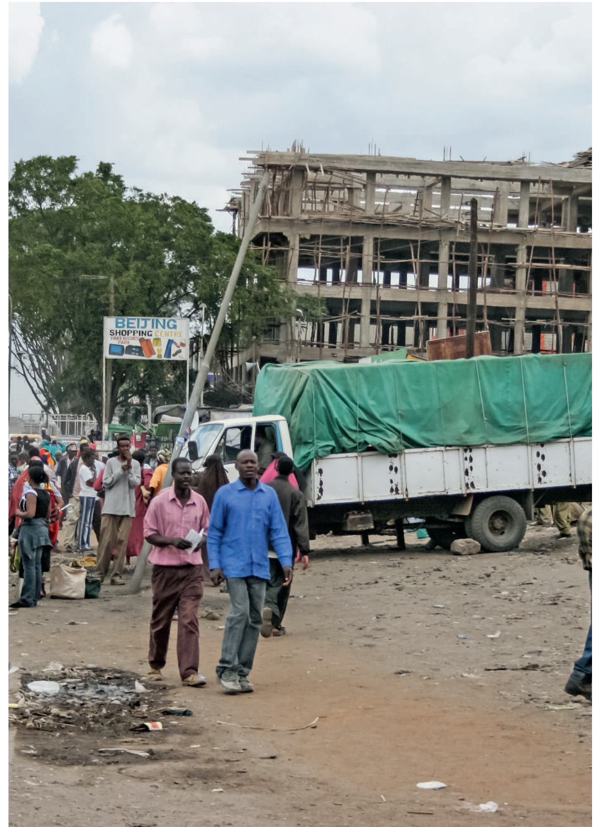
48 The new Beijing Shopping Centre under construction on First Avenue.
