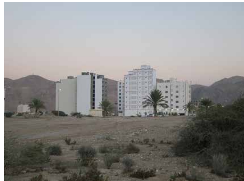
Commercial buildings in the Al Amarat plain
