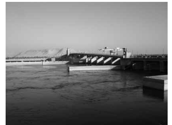
Barrage on the Nile River between Sohag and Qena, Egypt
