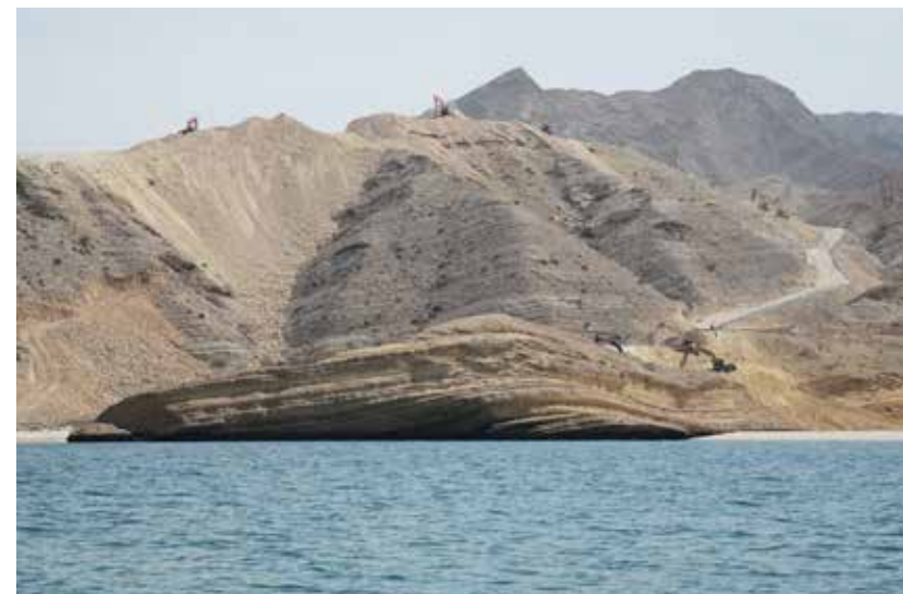
Construction for a coastal resort
