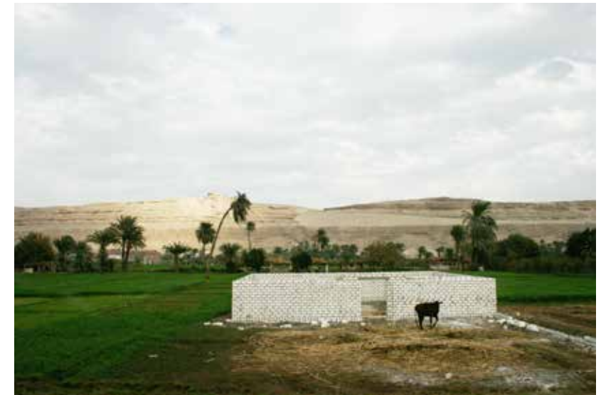
New construction on agricultural land
